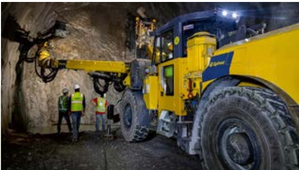
The work on the 125-kilometer Rishikesh-Karnaprayag Railway Line in the Himalayas is in full swing. The greenfield project has a total tunneling length of 218 kilometers. Here, Epiroc's automated and semi-automated machines, incl. the Boomer E2, are being used and contribute to increased efficiency on-site and reduced cycle time.
